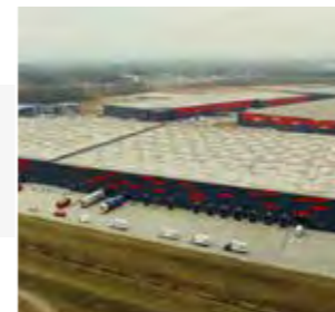
KOKOTÓW - Main warehouse
